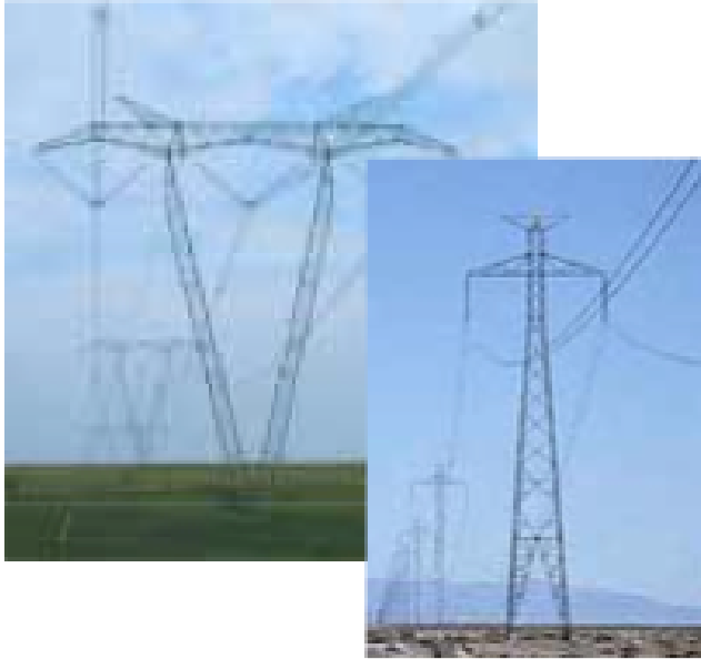
Fig 5. Transmission lines for 800 kV AC and 500 kV DC
